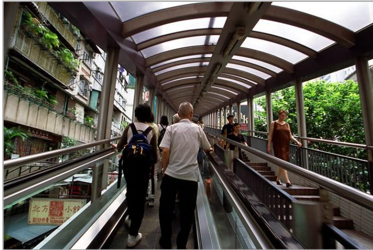
Central-Mid-Levels Escalator and Walkway System
