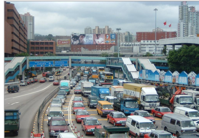
Approach roads leading to Cross Harbour Tunnel to Hong Kong
